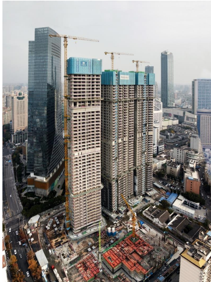
Aerial view of Center Residences under construction
