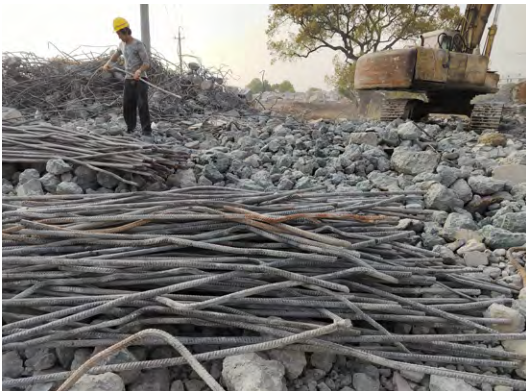
Dismantling temporary concrete bracing to recycle steel bar and concrete fragments in Westlake 66, Hangzhou
