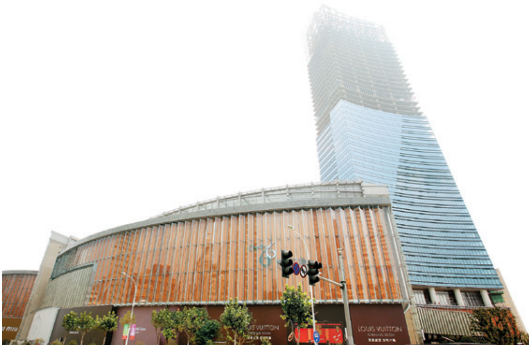
於二零一三年在無錫開業的恒隆廣場，突顯了本公司在建築設計上對最高標準的堅持 Opened in 2013, Center 66 exhibits the Company's commitment to upholding the highest standards of excellence in architectural design
