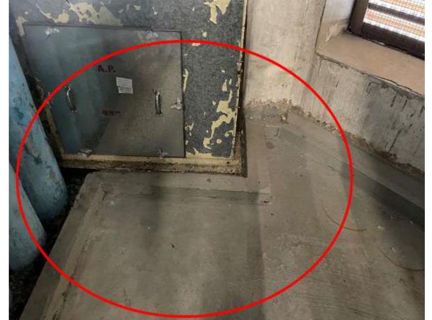
Example of an adaptation measure: Installation of a barrier between the airduct and chilled water pipe riser and external louver
