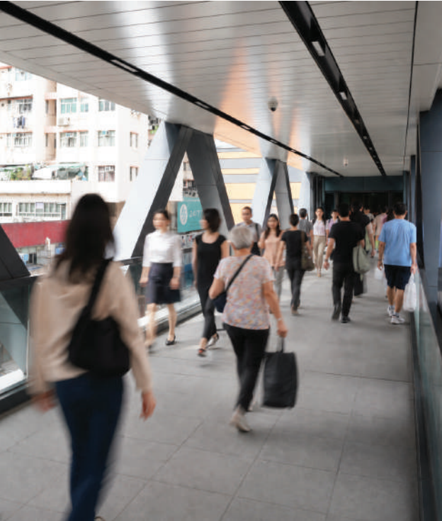
Already part of the daily routine for residents and office workers, the Amoy Footbridge is transforming the way people move through Kowloon Bay. 淘大天桥已成为九龙湾居民及上班族日常生活的一部分，正在改变人们穿梭九龙湾的方式。
