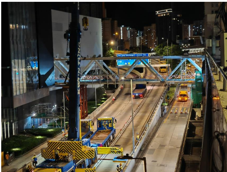
Photo 5: Amoy Footbridge under construction
