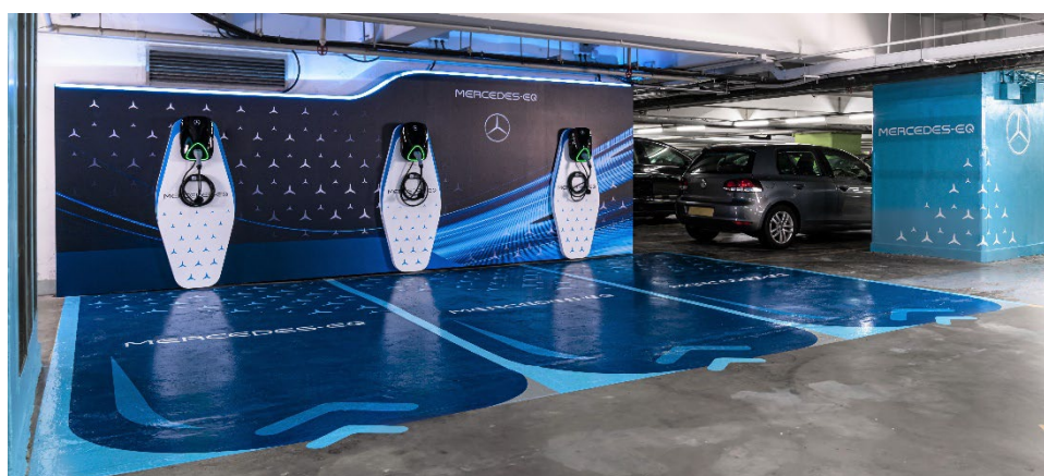
EV charging facilities at Kornhill Plaza, Quarry Bay
