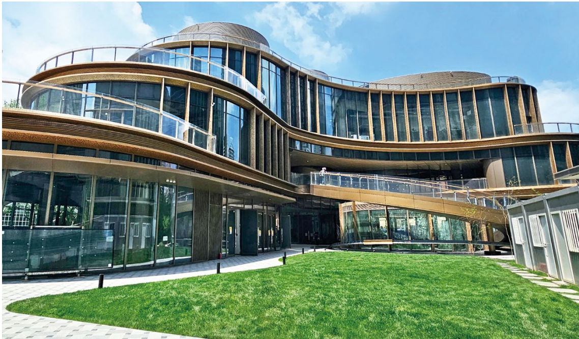
Exterior view of Plaza 66 Pavilion Expansion
