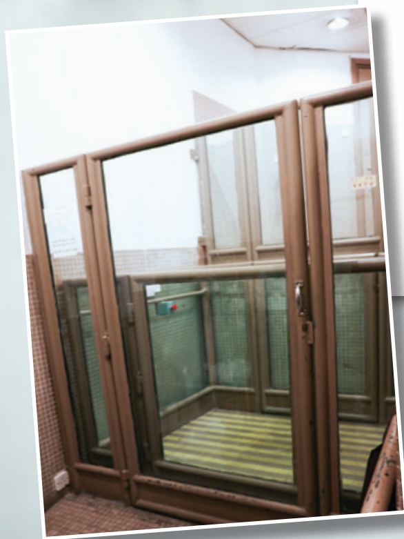
▲ 位於渣打銀行大廈的垂直升降台 The vertical lifting platform at the Standard Chartered Bank Building
