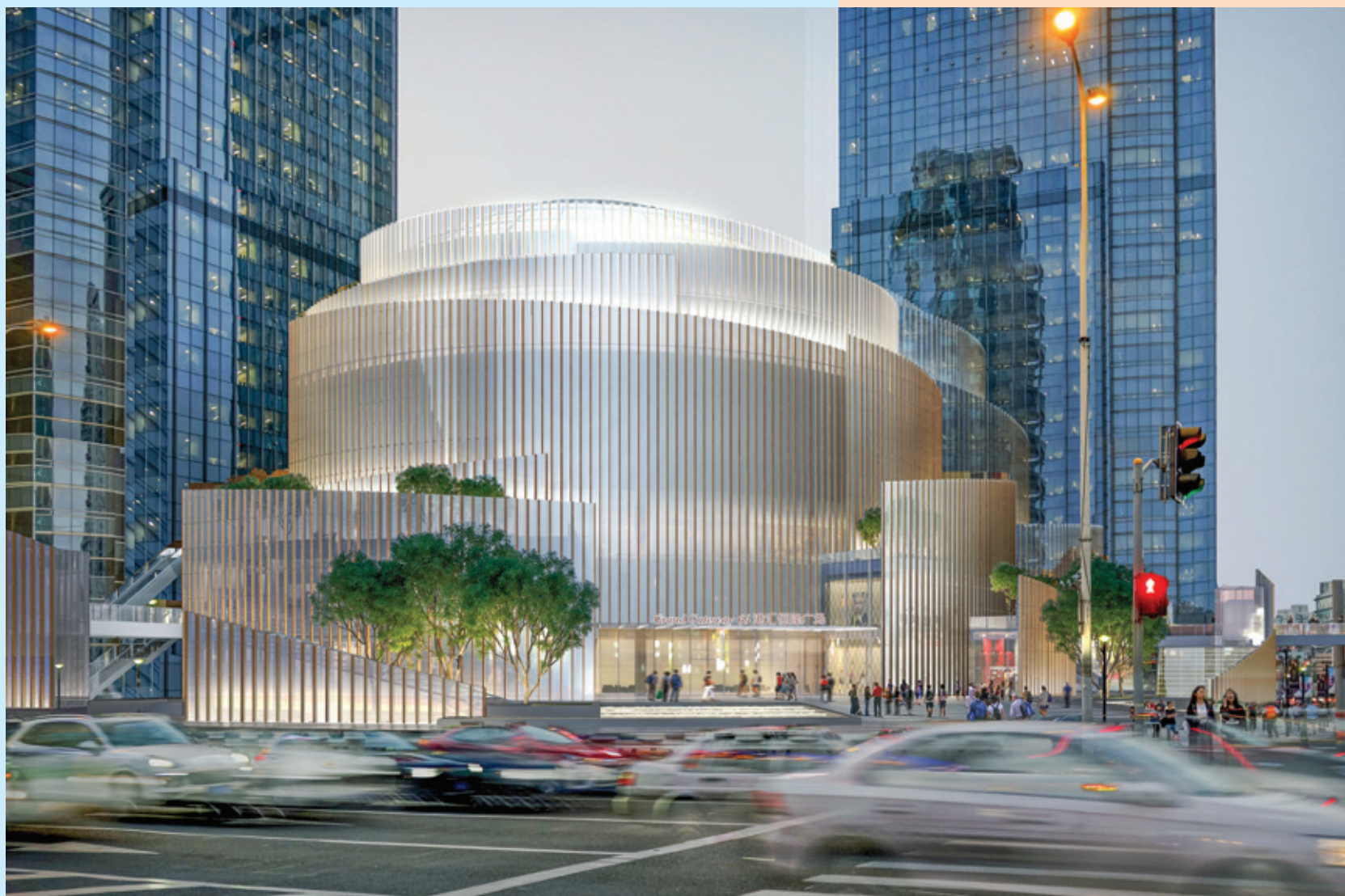
▼ 南座立面設計用上頂級玻璃與陶瓷嵌飾，獨具貴氣 The signature rotunda at South Building was re-designed and clad with elegant glazed panels and terracotta inlays
