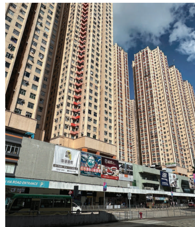
Since their completion in the 1980s, Amoy Gardens and Amoy Plaza have witnessed Kowloon Bay’s shift from an industrial district to an everyday community hub. 自八十年代落成以來，淘大花園與淘大商場一直見證九龍灣由工業區走向社區生活樞紐。
