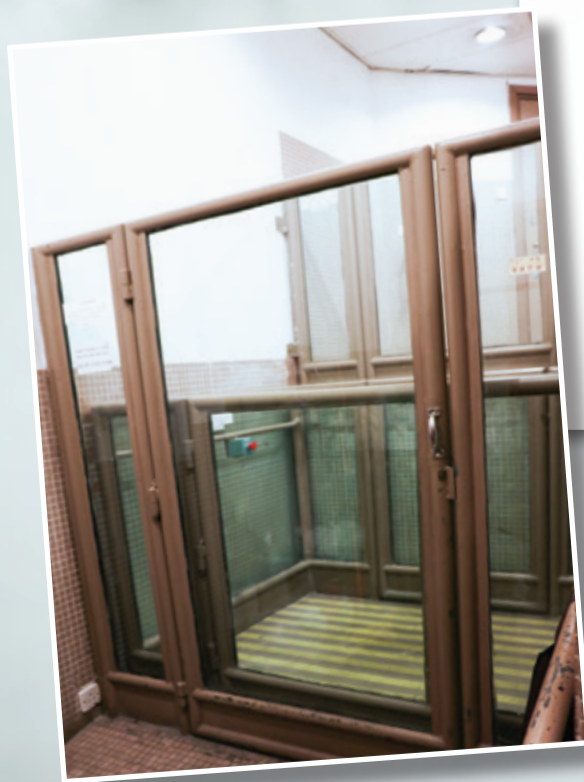
▲ 位于渣打银行大厦的垂直升降台 The vertical lifting platform at the Standard Chartered Bank Building
