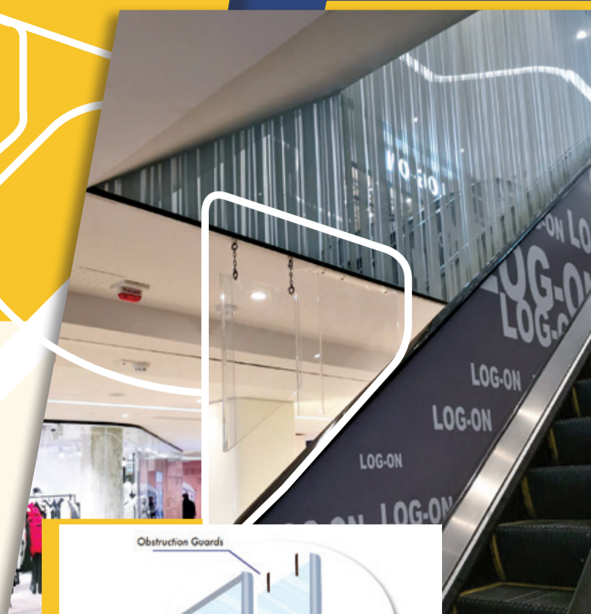
▲ Fashion Walk扶手电梯的防护挡板 A fixed and suspended guard installed for one of Fashion Walk's escalators
