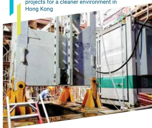
An advanced battery energy storage system has been introduced to replace traditional diesel generators at our new development projects for a cleaner environment in Hong Kong
