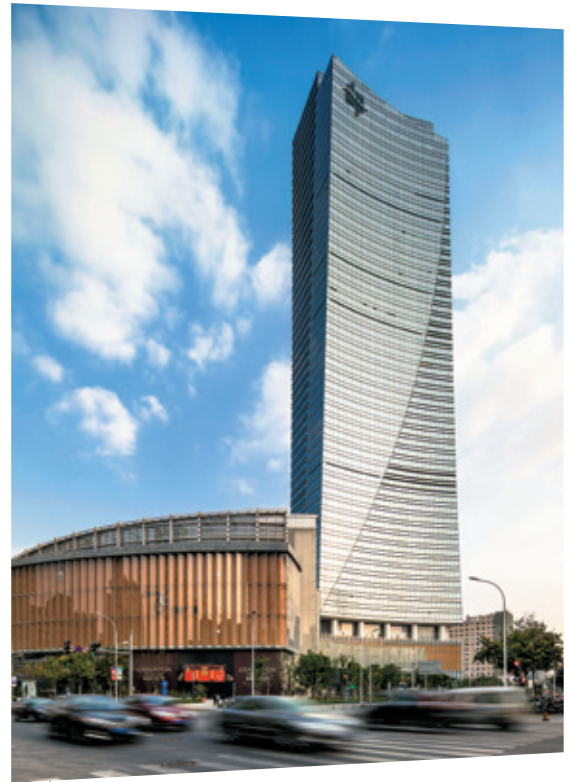
Center 66 – Phase 1 & 2 will be the largest retail and commercial landmark in the central business district of Wuxi
